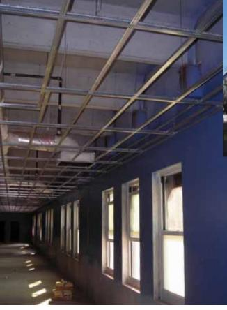
Suspended drywall below the shallow depth of the precast concrete double tees provided a finished ceiling on each level.
